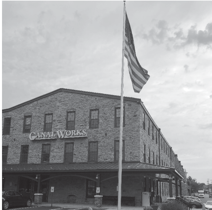
Canal Works - New Administrative Offices
